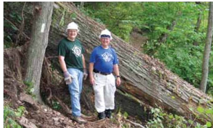
A huge blowdown dictated moving the footpath of the A.T. just south of the James River by members of the NBATC, including Bill Bishop (left) and Joe Chavez (right).
