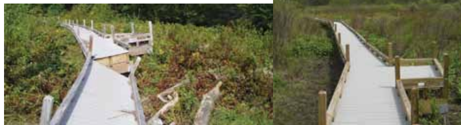
Thundering Falls Boardwalk before and after repairs. Photo courtesy of the Green Mountain Club
