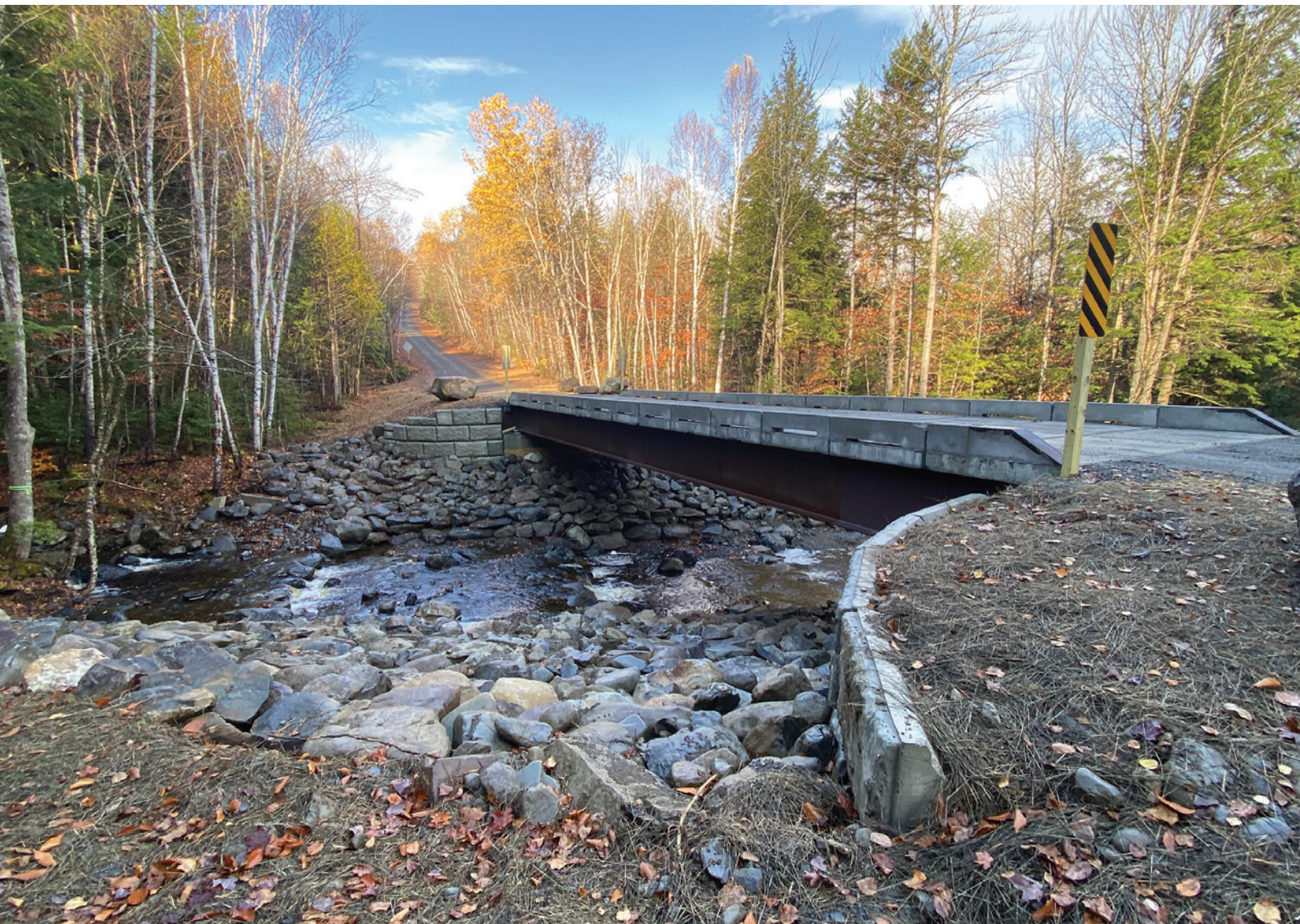
IMMEDIATELY AFTER THE 70-FOOT-LONG STEEL AND CONCRETE CLEAR-SPAN BRIDGE WAS INSTALLED IN THE SUMMER OF 2023, FISH BEGAN PASSING UNDERNEATH IT. (ABOVE RIGHT) PROJECT PARTNERS, FROM LEFT: PETE RUKSZNIS, MAINE DEPARTMENT OF MARINE RESOURCES; STEVE TATKO, APPALACHIAN MOUNTAIN CLUB; AND MARIAN ORLOUSKY, ATC. Photos below and above left by Leah Beck
