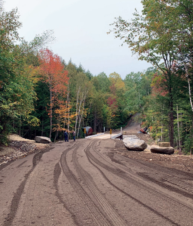
IMMEDIATELY AFTER THE 70-FOOT-LONG STEEL AND CONCRETE CLEAR-SPAN BRIDGE WAS INSTALLED IN THE SUMMER OF 2023, FISH BEGAN PASSING UNDERNEATH IT. (ABOVE RIGHT) PROJECT PARTNERS, FROM LEFT: PETE RUKSZNIS, MAINE DEPARTMENT OF MARINE RESOURCES; STEVE TATKO, APPALACHIAN MOUNTAIN CLUB; AND MARIAN ORLOUSKY, ATC. Photos below and above left by Leah Beck
