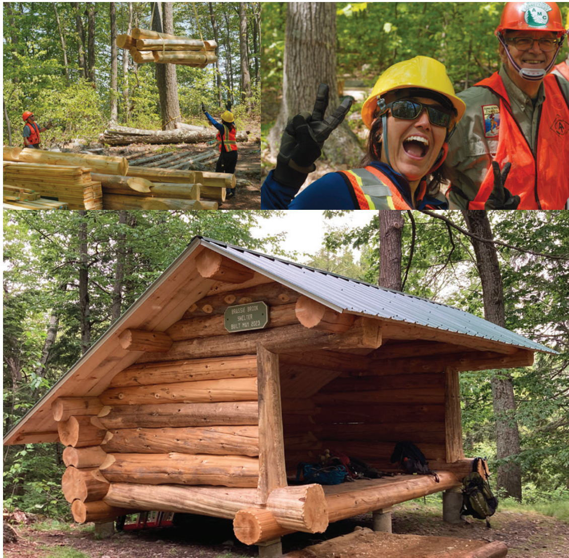
Constructing the new Brassie Brook shelter in Connecticut required a dozen airlifts of logs, roofing, and other materials. The effort involved in coordinating the project resulted in jubilation upon the safe delivery of shelter components. The shelter opened in May 2023. Photos by Christoph Geiss
